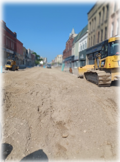
Stage 2 Roadway Prep
